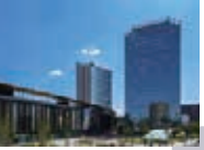
Beijing FA Center MITSUBISHI ELECTRIC AUTOMATION (CHINA)LTD.
