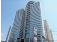
Thailand FA Center MITSUBISHI ELECTRIC FACTORY AUTOMATION (THAILAND) CO.,LTD
